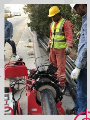
HDPE (High Density Poly Ethylene) are jointed by butt fusion process.
